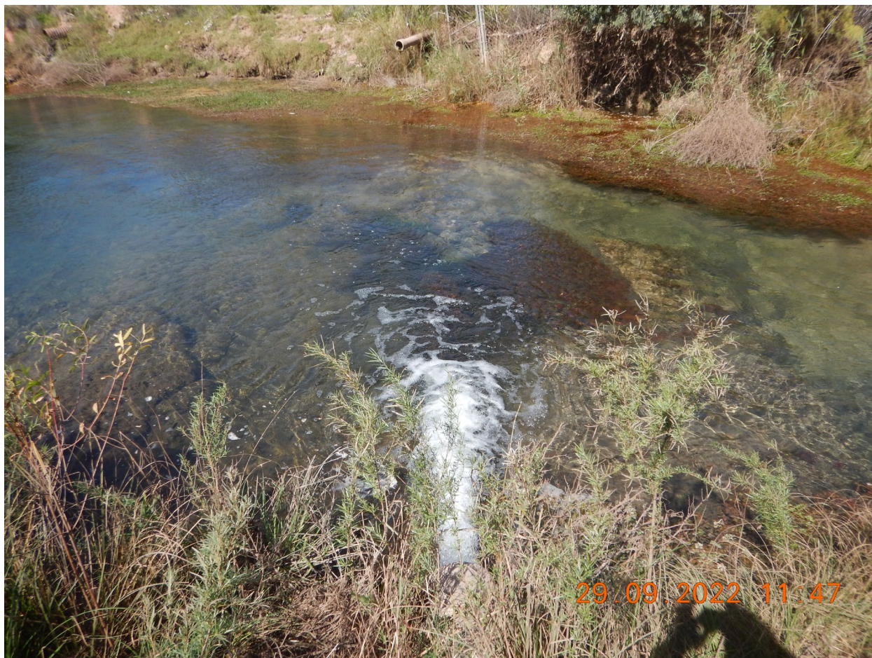
View of WWTP's outfall discharge into El Rito Creek. (DSCN2363) Photographed by D. Esparza.
