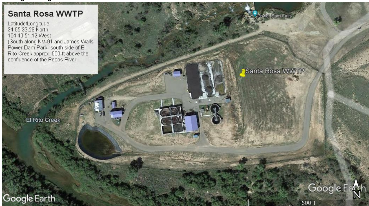
Aerial Image #1: Overall view of the City of Santa Rosa Wastewater Treatment Plant
