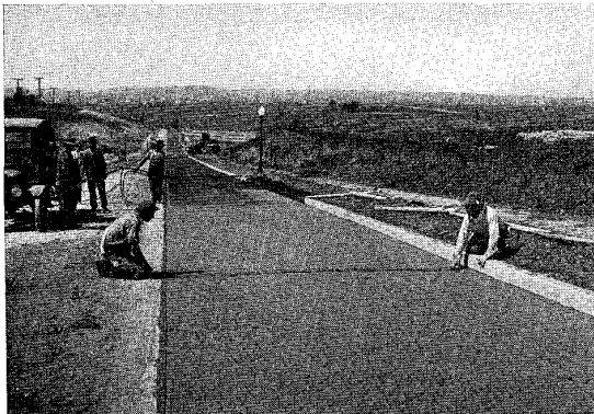
CONCRETE IN STREETS OF MONTE MAR VISTA TRACT, LOS ANGELES, CALIF., CURED BY "HUNT PROCESS" USING "McEVERLAST" PRODUCT
