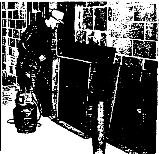
Vent stack flashings and shower pans are made with 6-lb. sheet lead with all joints lead burned. Precast shower receptors are then placed within the lead pans as at left, below.
