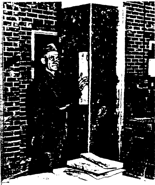
The X-ray room is lead-lined with 6-lb. sheet lead. The supporting columns are wrapped with sheet lead and walls are made with cinder block lead sandwiches.
