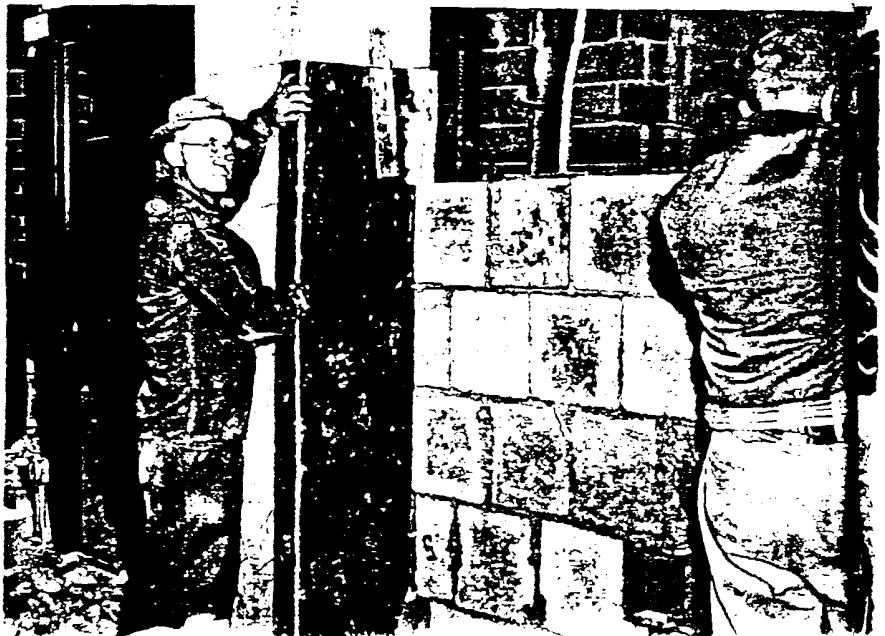
The X-ray room is lead-lined with 6-lb. sheet lead. The supporting columns are wrapped with sheet lead and walls are made with cinder block lead sandwiches.
