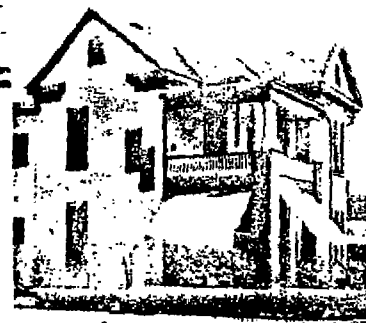
Baton Rouge home finished inside and out with Sherwin-Williams products — another job Sherwin-Williams helped the painting contractor to close. Products used: SWP House Paint for body and trim; S-W Screen Enamel; S-W Porch and Deck Paint; S-W Ruxper and Mar-Not Varnish. No matter what surface needs paint—Sherwin-Williams makes the right paint for it.
