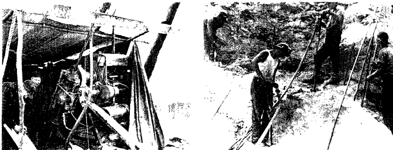
Left. One of the rotary core drills for proving deposits in the asbestos quarry. Right. Men at work with hand-operated compressed air drills preparing blast holes
