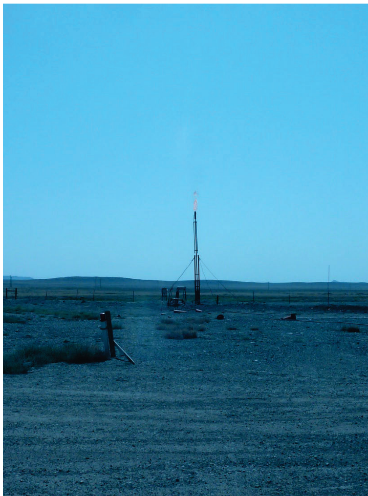
Photo of Production Flare
