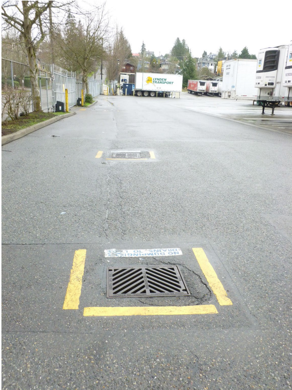
Photo 1 / P1010174 – Catch Basin Line, facing east
