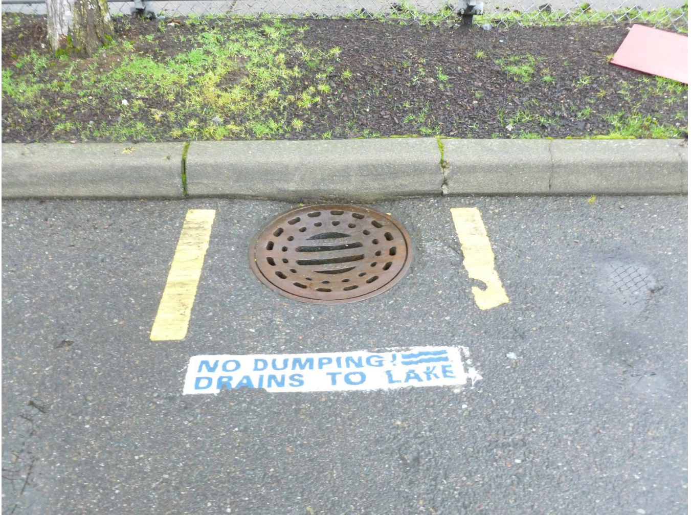
Photo 3 / P1010176 – Catch Basin, Type 2, facing north
