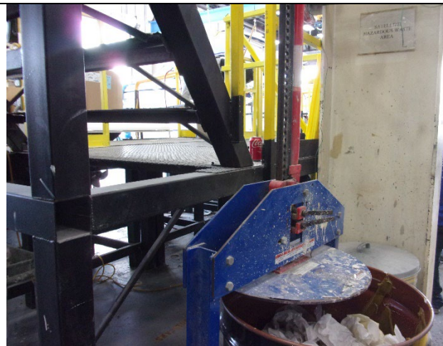
Figure 16: 12:26 PM Building G Picture one of two opened 55-gallon SAA containers observed.
