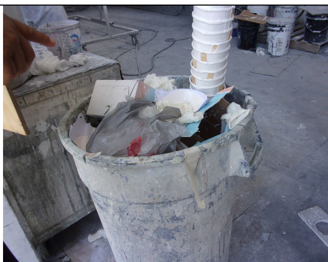
Figure 28: 1:07 PM Commodore Building Lamination One 45-gallon container observed opened with accumulated material.
