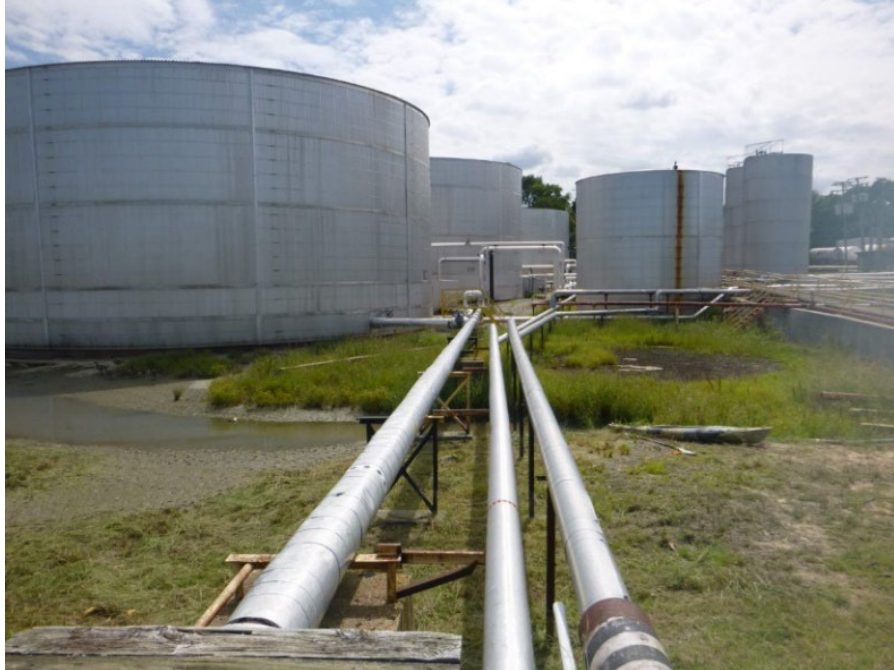
Photograph 3. Bermed Diversion Pond at Tank Farm (Smaller basin)
