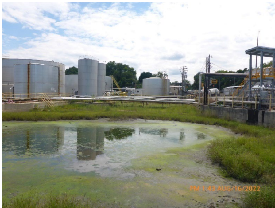
Photograph 2. Bermed Diversion Pond at Tank Farm IU Sampling Point for Outfall H-8A
