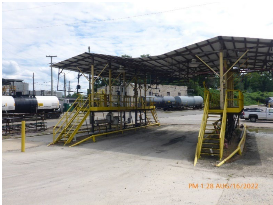
Photograph 1. Truck Washing Bay - Outfall H-8
