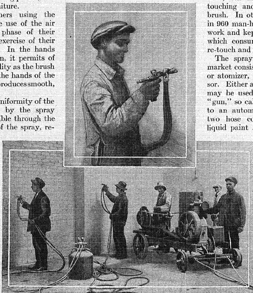
Upper: Air Brush in Operation. Lower: Complete Spraying Outfit with Two "Guns"
