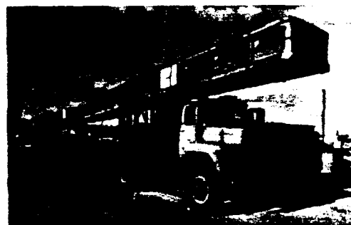
A desalting plant in Key West, Florida, received in 1971 the longest welded titanium tubes ever produced. Fabricated at TIMET, these 105-foot titanium tubes combat the corrosive effects of sea water in the process of converting salt water to fresh water.
