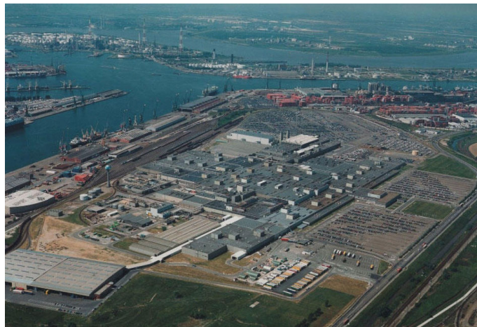
The Opel plant in Antwerp, before site clearance. © Opel
