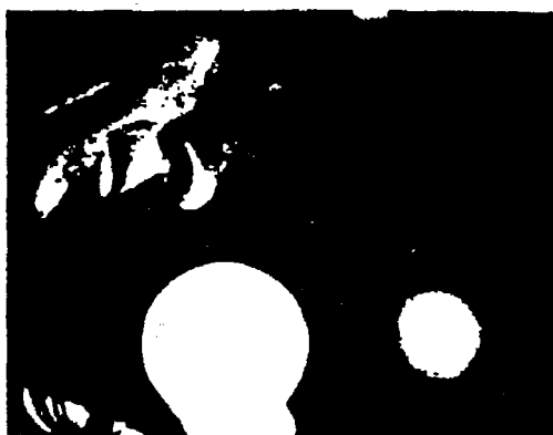
Marvin Pipkin of Nela Park compares the even diffusion of "Soft White" lamp, on left, with standard frosted lamp on same wattage, on right.
