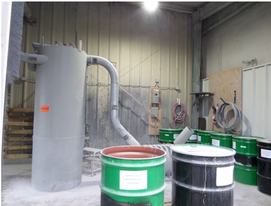
Photograph 2: Vacuum Unit Room, Seven Empty Containers, Two Drums of Sanding Waste, Dust Has Accumulated on the Floor
