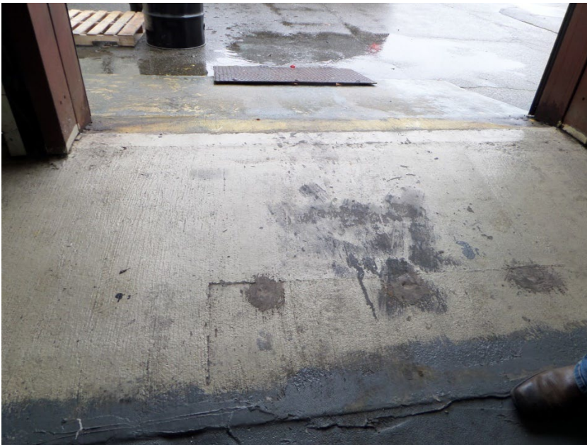
Photograph 22: Interior Picture of CAA Showing Raised Entrance Slope
