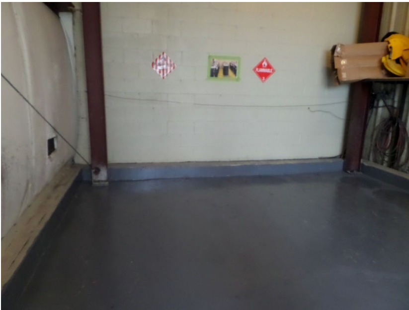
Photograph 21: Interior of the CAA.
