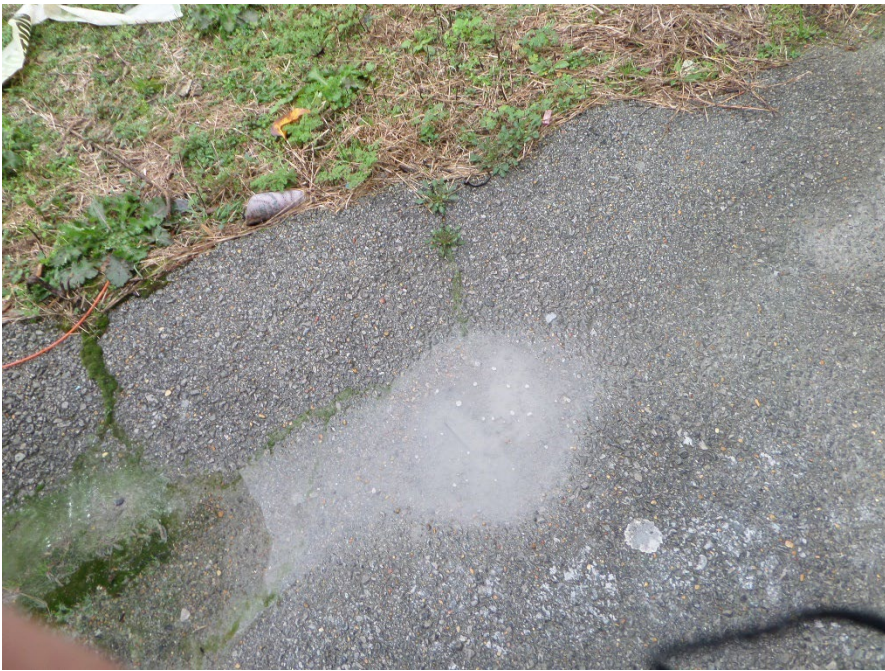
Photograph 5: Outside of Vacuum Dust Room
