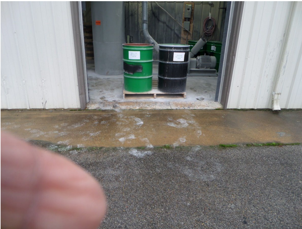
Photograph 7: Dust on the Floor and Exterior of the Vacuum Dust Room
