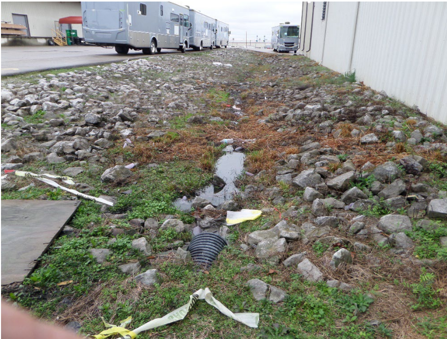
Photograph 4: Drainage Ditch Outside of Vacuum Unit Room
