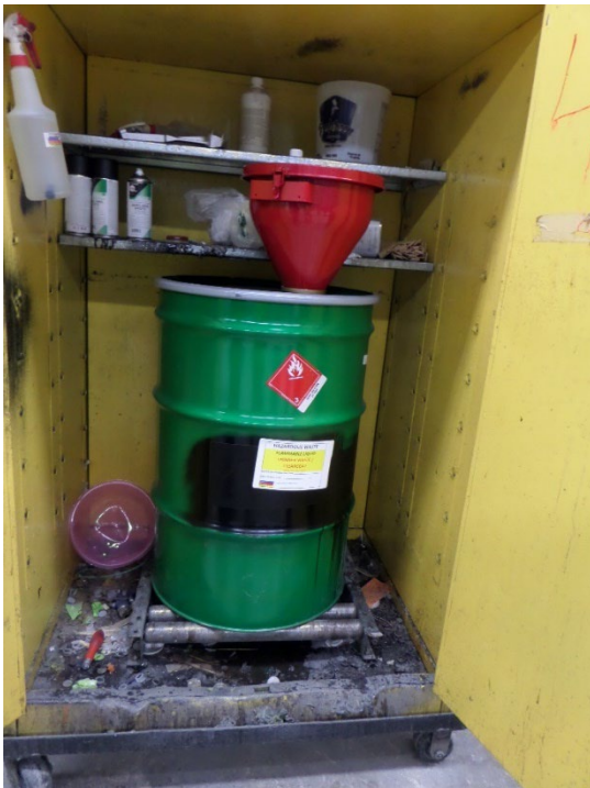
Photograph 12: SAA HW Drum Properly Labeled as Hazardous Waste and Hazard Marking
