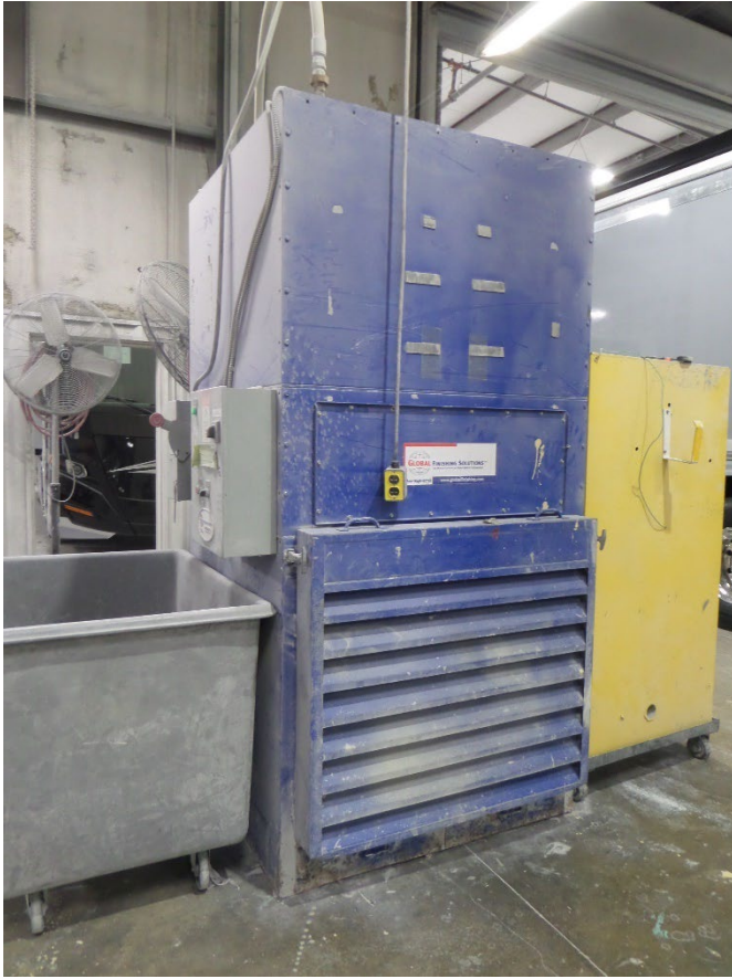
Photograph 1: Component of Dust Vacuum Unit in the Sanding Building
