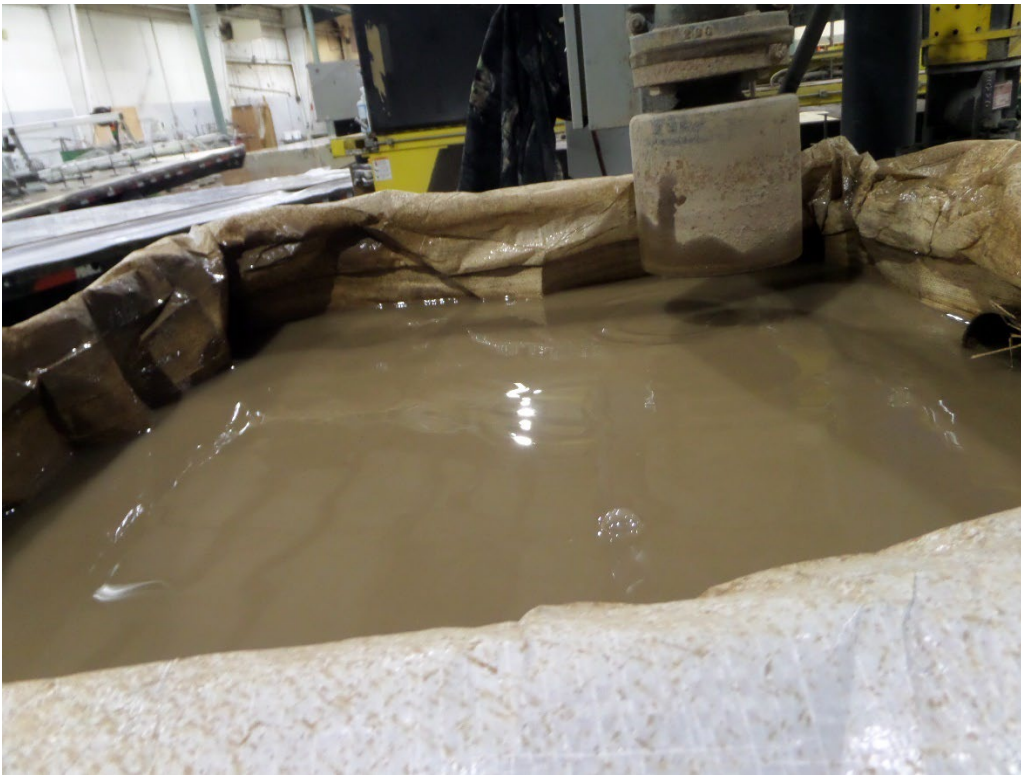
Photograph 9: Water & Sludge in the Tile Building
