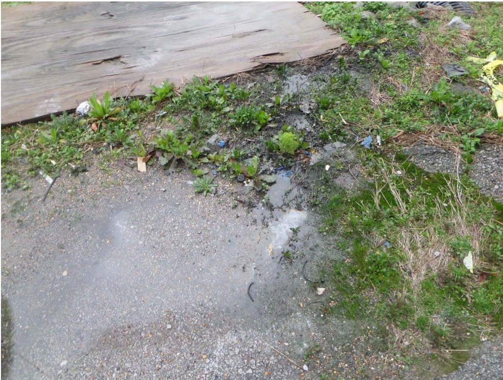
Photograph 6: Outside of Vacuum Dust Room
