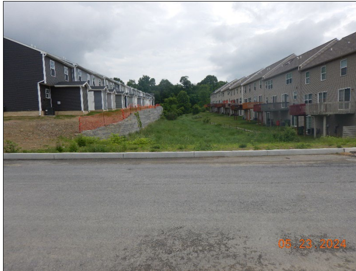
Terrace at Maplewood Date: 23 May 2024 Photo ID: DSCN5385.JPG Photo taken by: Katelyn Almeter Notes: East facing view of drainage area between two rows of townhouses.
