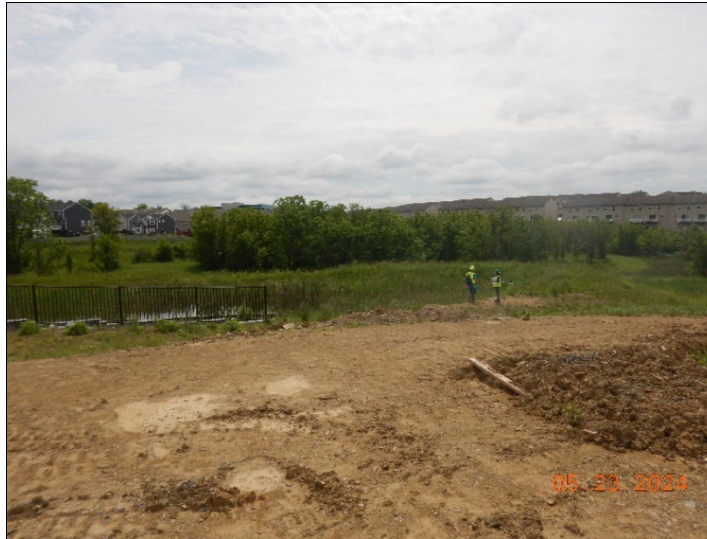
Terrace at Maplewood Date: 23 May 2024 Photo ID: DSCN5394.JPG Photo taken by: Katelyn Almeter Notes: Overview of construction area.
