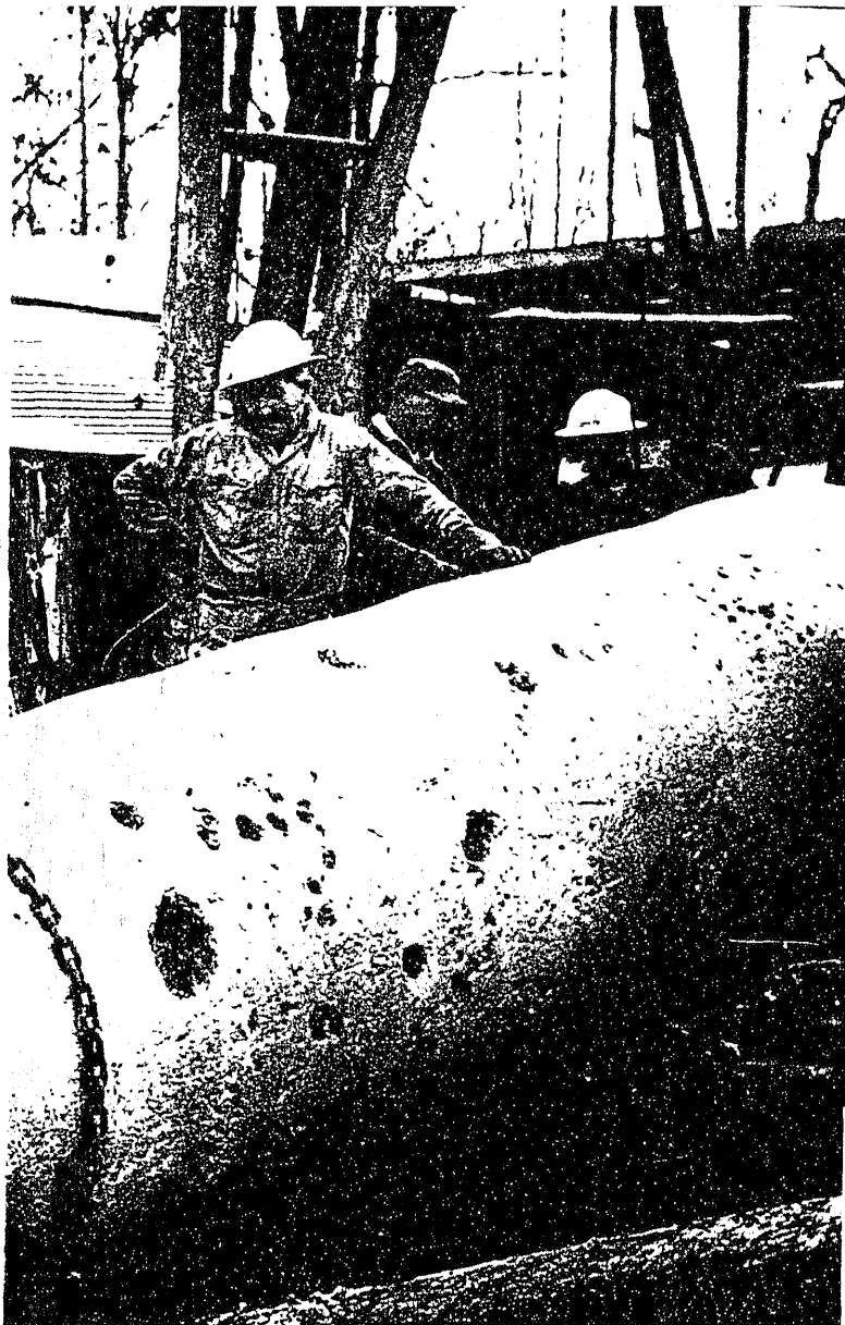
Shaft-sinking with big drill cuts 52-in. core at Viburnum
