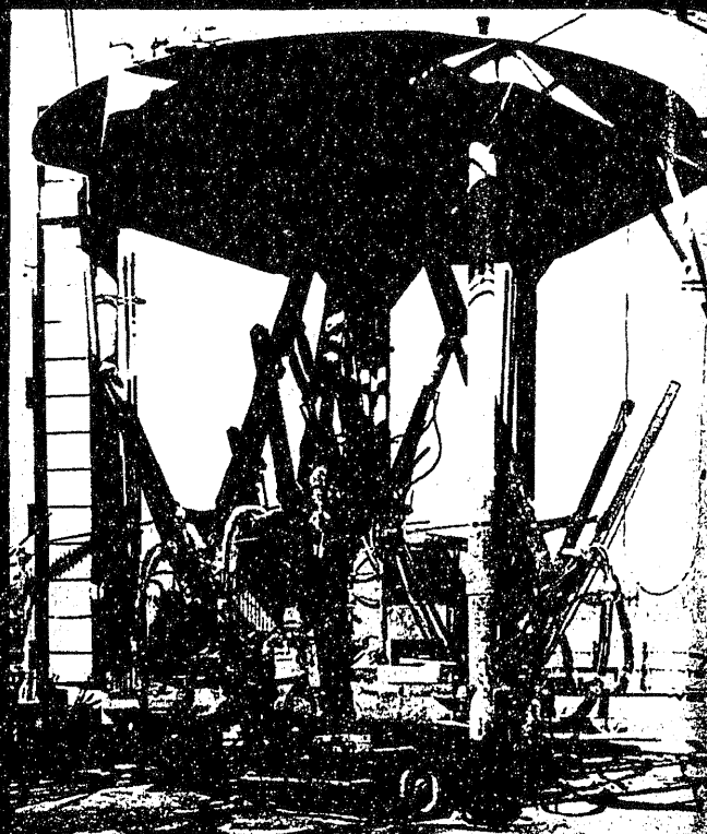
Shaft-sinking at Pea Ridge is done faster with this drill jumbo mounted on sinking cage
