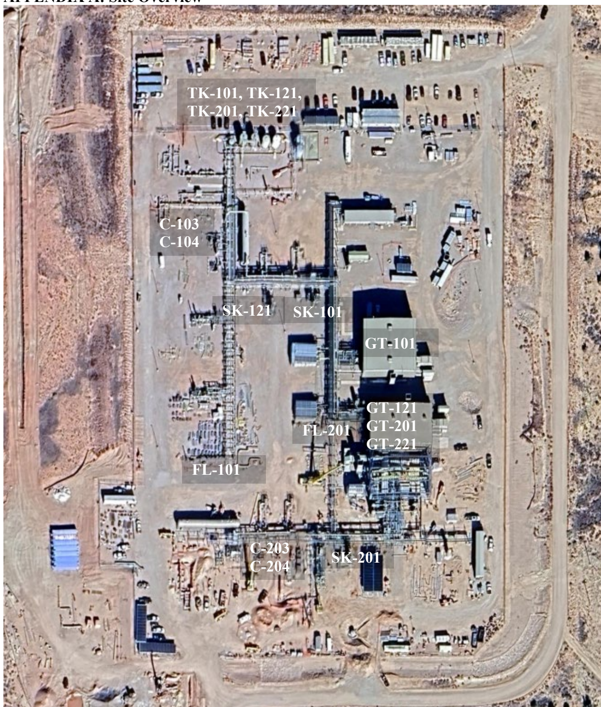
Figure 1: Walker Hollow Compressor Station Aerial View
