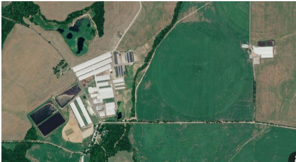
Photo 1: Aerial photo, sourced from Google Earth, depicting the facility and surrounding areas.
