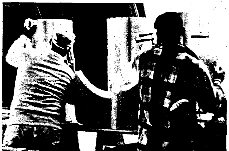
Members of the Asbestos Workers Union install pipe covering in Oyster Creek generating station now being built at Toms River, N. J. Site was visited by IHRP team. (See story on page 8)
