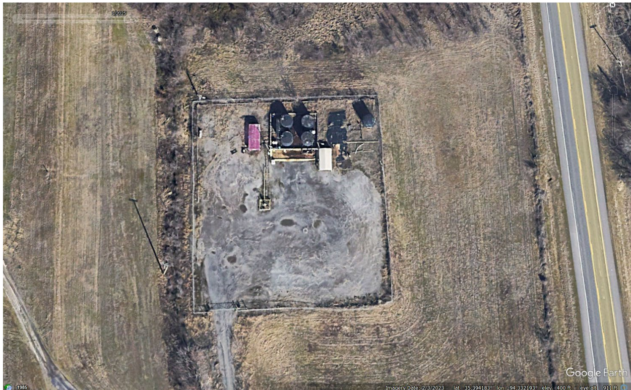
Map 1. Aerial imagery (Google Earth dated 02/03/2023) of the Capstone Oilfield Disposal of Arkansas, LLC / Bohannon No. 4 SWDS Tank Battery.
