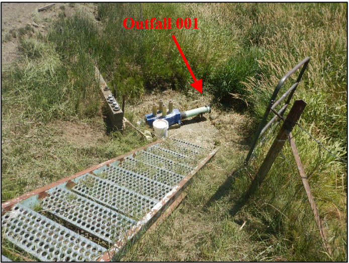
Photograph #18 (DSCN9162) Description: View of the Facility's Outfall 001 to John Dobb Creek.
