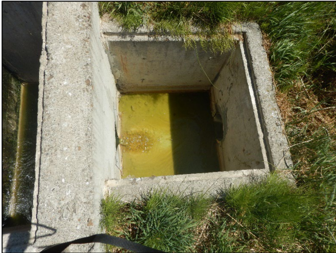
Photograph #09 (DSCN9139) Description: Additional view of the Facility's v-notch weir.
