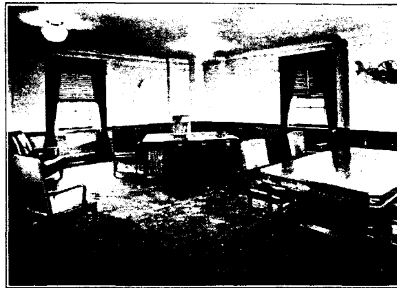
One of the lovely private offices in the Federal Court House decorated with pure white lead paint.
