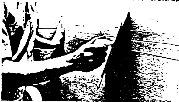
Simplified, wrinkle-free attachment of self-stick Type P IMPERIAL Tape speeds joint reinforcing, boosts production.
