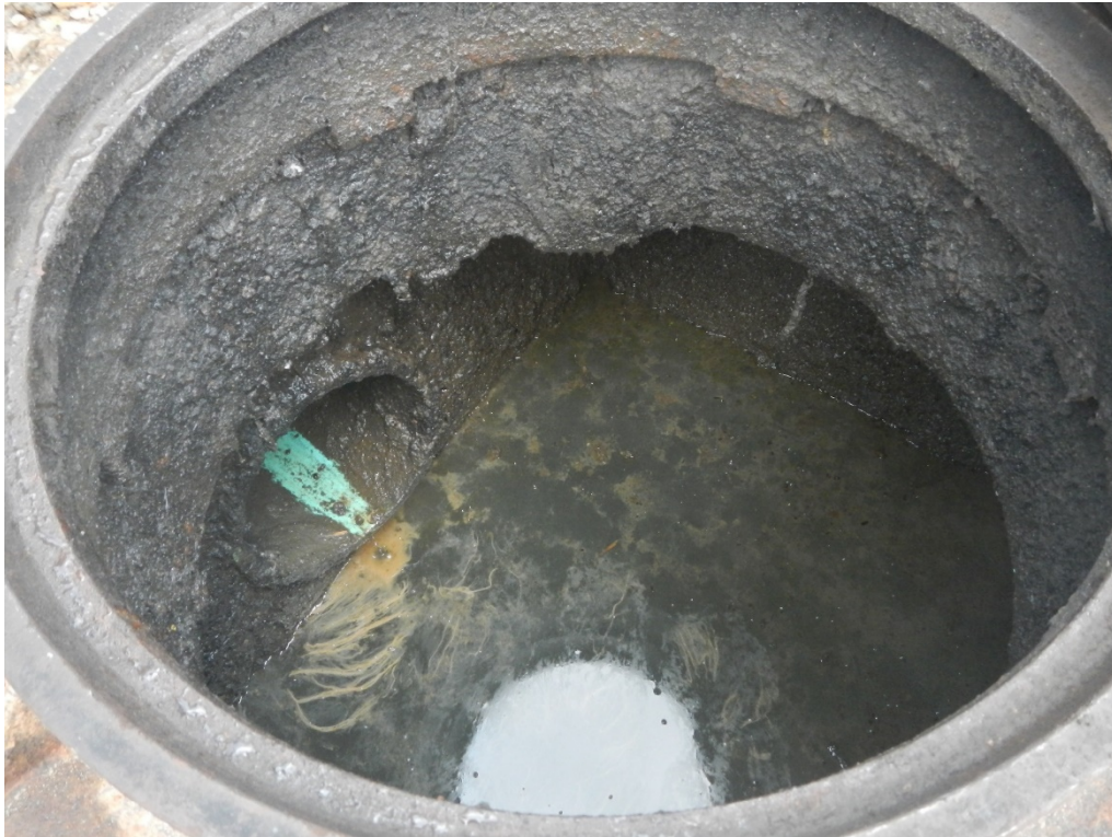
Photo 1 Inside of oil and grease separator 1.
