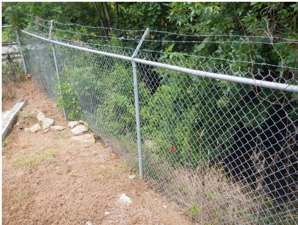
Photo 6 Actual location of discharge for outfall 002. Effluent pipe is located behind brush and discharges directly into Town creek (Downstream of other facilities and Brownfields)
