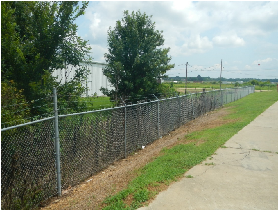
Photo 8 Chainlink fence showing distance from actual discharge point to sampling point. Distances between fence posts are estimated at 10 feet. For 22 segments this shows that the sampling point is located 220ft downstream of discharge point.
