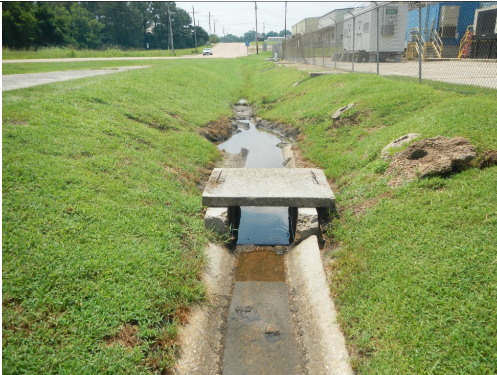
Photo 3 Sampling site for outfall 1. Area receives effluent from neighboring facilities.
