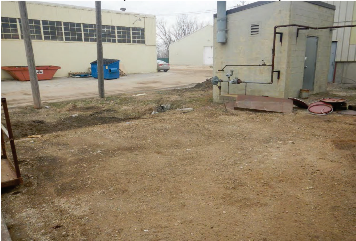
Photo 16, MS4 open ditch 30 feet from the collection system
