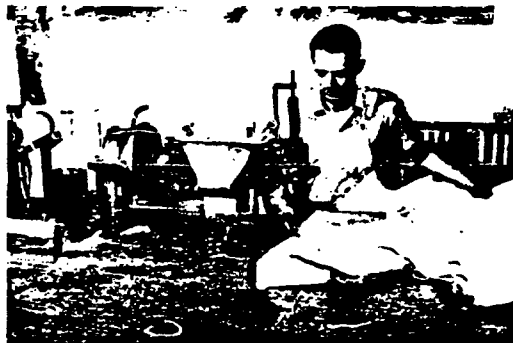
SLICK STITCH —"Just a little thing I ran up myself," says John Jones as he stitches together the various pieces of a custom-tailored turbine-blanket section. The machine he uses is a heavy-duty job that stitches with heavy wire covered with asbestos. The "thread" must pass through a lubricating bath before it can be used to sew the heavy asbestos-jacket pieces.
