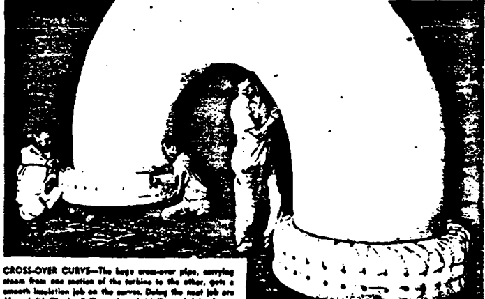
CROSS-OVER CURVE —The huge cross-over pipe, carrying steam from one section of the turbine to the other, gets a smooth insulation job on the curves. Doing the neat job are (from left) Charles Sullivan, Joseph Mullin and John Jones.
