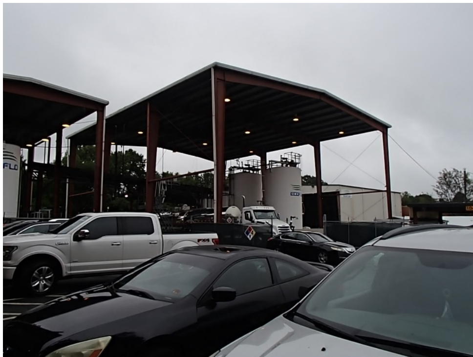
Photo 2: View of ECOFLO's facility from the street.
