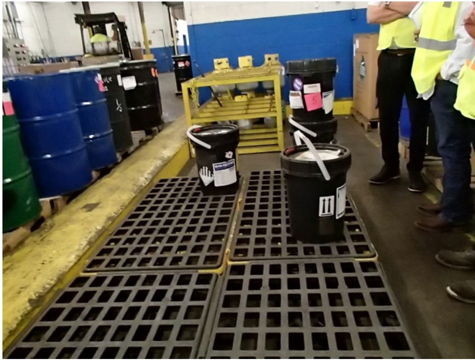
Photo 3: View of 4 PCB 5-gallon containers on a containment pallet in the PCB Storage Area.
