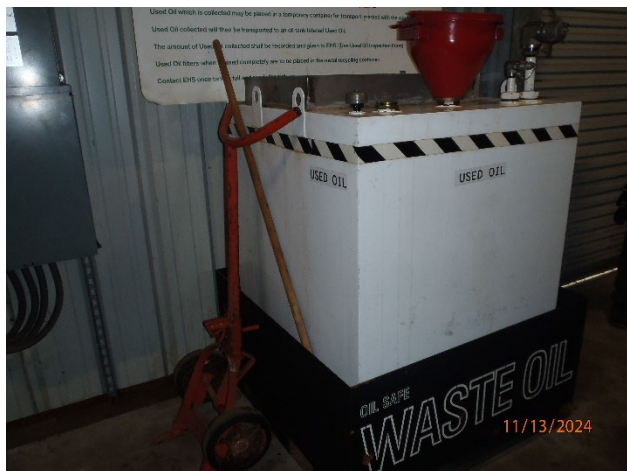
Picture 15 – Spinning Maintenance Used Oil tank
