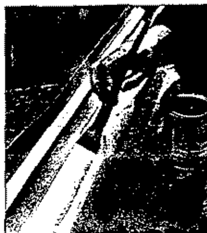
Adhesive bonding of the flap is recommended for cold- and dual-temperature lines. Armstrong 520 Adhesive forms a vaporproof seal.
