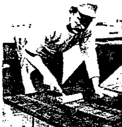
When Armaflex Sheet is used with full adhesive coverage, adhesive is easily applied with brush or roller.
