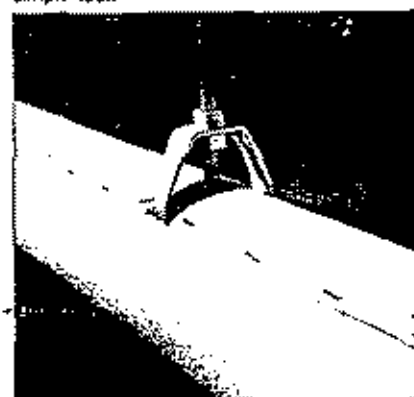
Finished installation around clevis hanger is neat and workmanlike.
