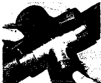
Fitting covers are easily assembled from miter-cut pieces of pipe insulation. For larger sizes, special template patterns are available for cutting covers from Armaflex Sheet.
