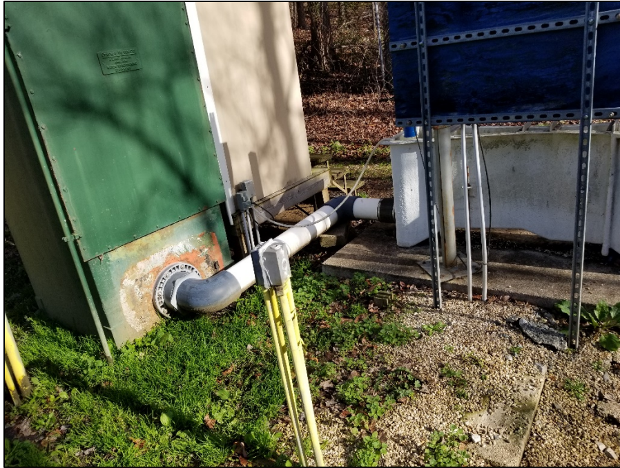
Photograph 9. View of the effluent end of the green rectangular filter unit. Plant representatives were unsure of the media in the unit or its exact treatment function.
