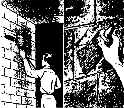
Apply neutralizer with mop or brush. Allow to dry.
