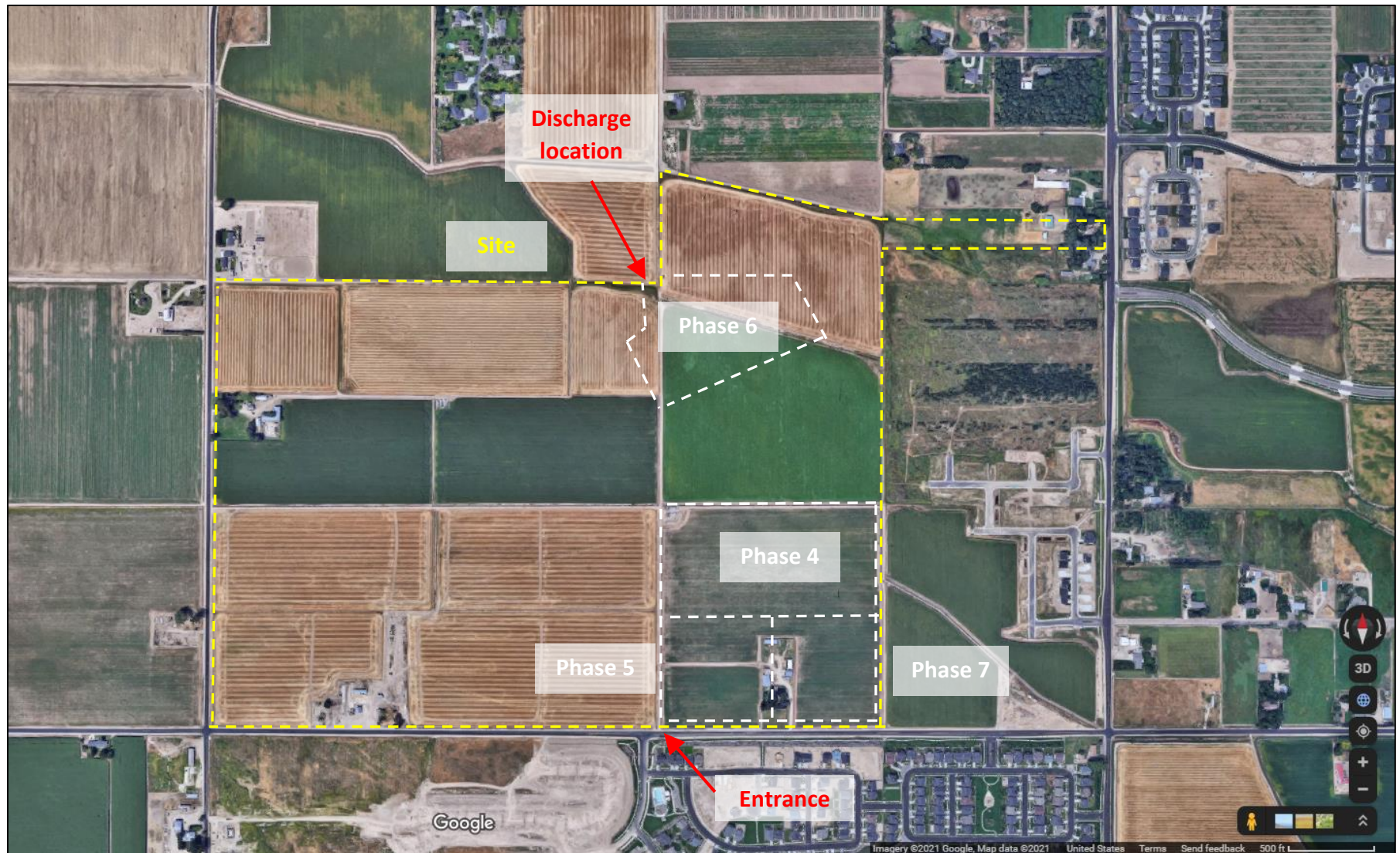
Exhibit 1. Google Maps image (copyright date: 2021). Location of The Oaks North in Meridian, Idaho. Note the approximate Site perimeter outlined with the dotted yellow line, the approximate Phase perimeters outlined with the dotted white line, the discharge location, and the entrance.
