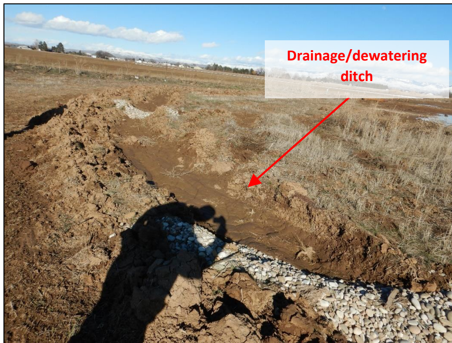
Photograph 14. View, facing northeast, of a drainage/dewatering ditch observed in Phase 6. Rock check dams had been installed along the length of the ditch.
