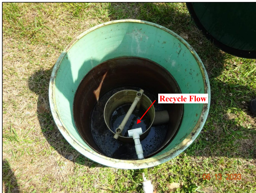
Photograph 7. View into the second opening of the primary tank. Note the white plastic recycle flow pipe at the edge of the opening.
