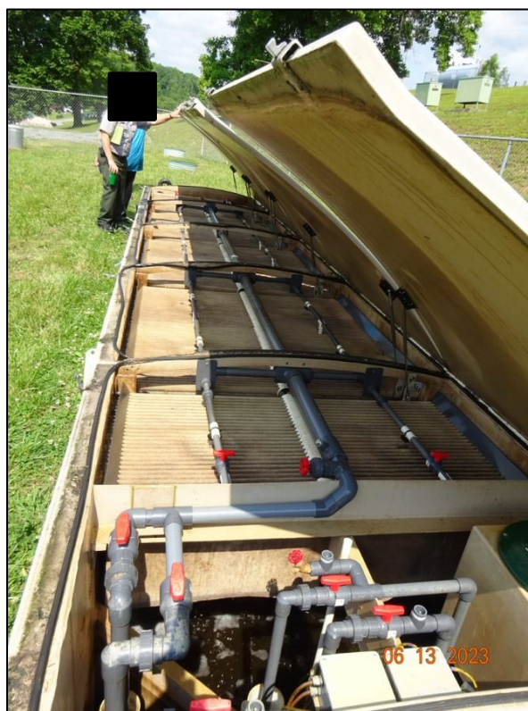
Photograph 8. View, facing west, of the Orenco AdvanTex® recirculating media filter.
