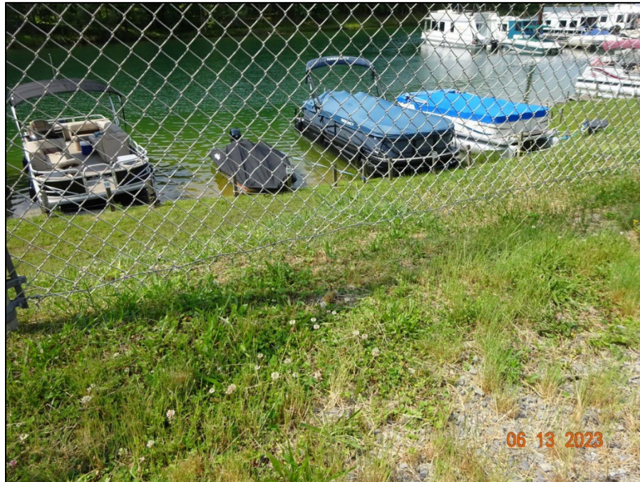
Photograph 15. View, facing south, of gap in plant perimeter fencing.
