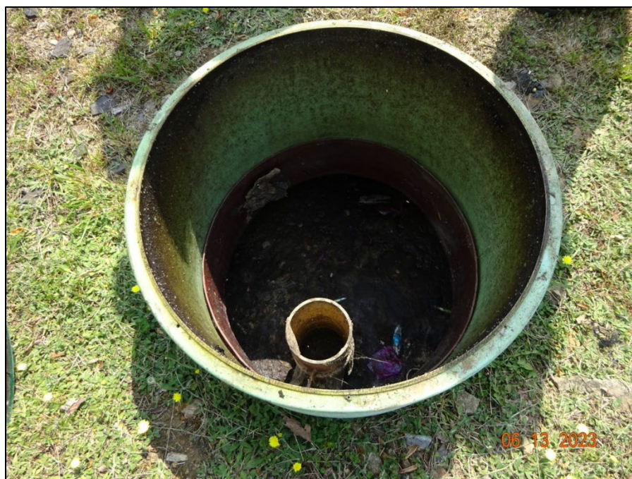
Photograph 6. View into the first opening of the primary tank. Note some trash and floating debris.
