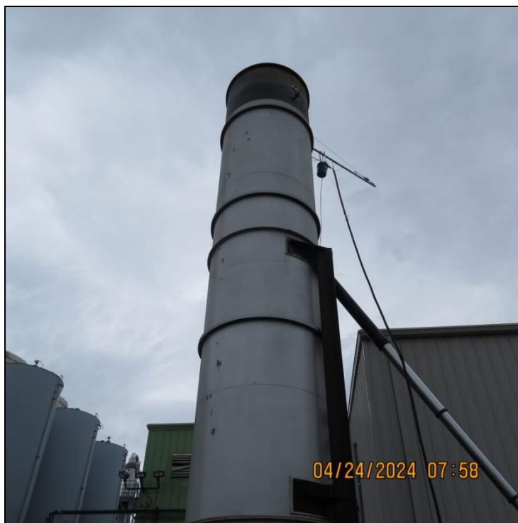
Photograph 1: Temporary Thermal Oxidizer Stack
