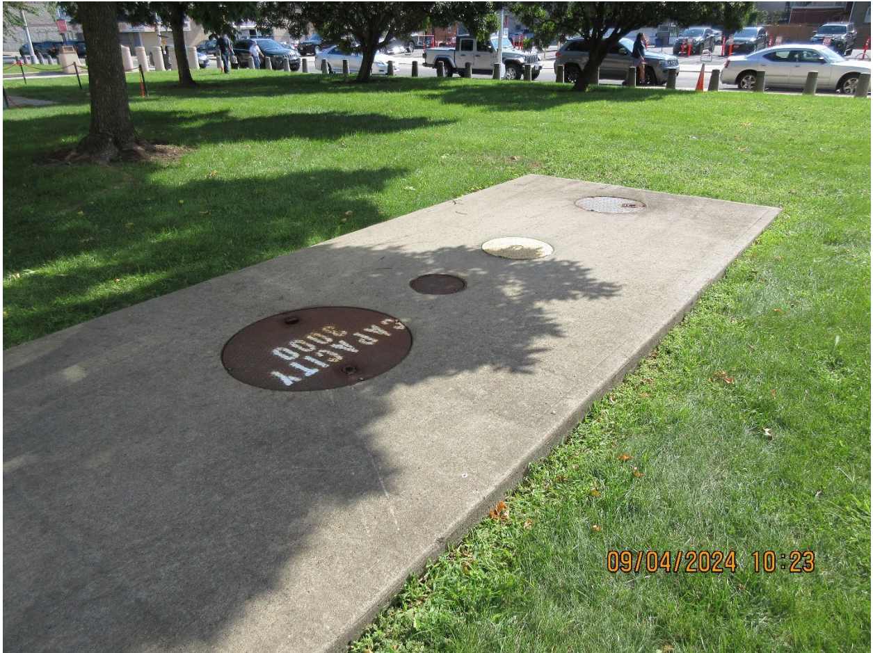
Photo 1 – Sumps for UST facing Mulberry Street
