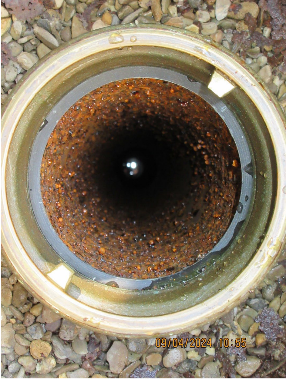
Photo 10 – Access port pipe interior
