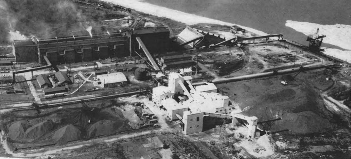
Aerial view of Q.I.T. operation at Sorel, Quebec. The electric furnace plant appears in the background and the new pre-treatment plant in the foreground.
