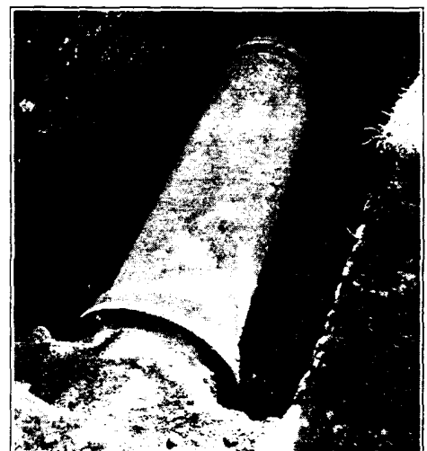
← Cast iron water pipe with cast lead joints laid in 1817 in Philadelphia.
