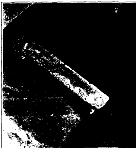
← Cast iron water pipe with cast lead joints laid in 1817 in Philadelphia.
