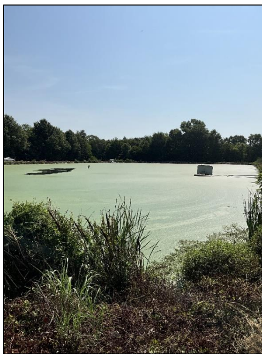
Photo 4: Cell 1 (location of non-functional aerators)
