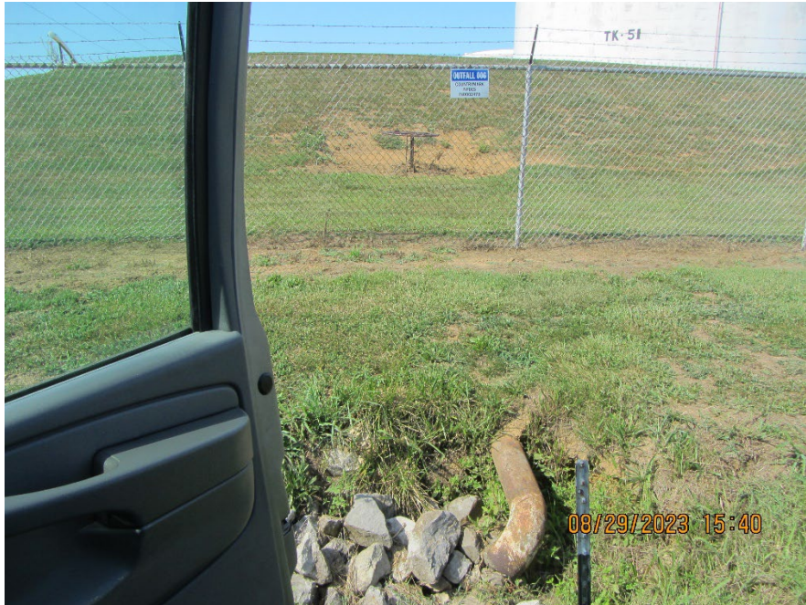
26: IMG_0346 Description: Outfall 006 Location: Northwest side of the Facility Camera Direction: North Date/Time: 8/29/23, 3:40 p.m.
