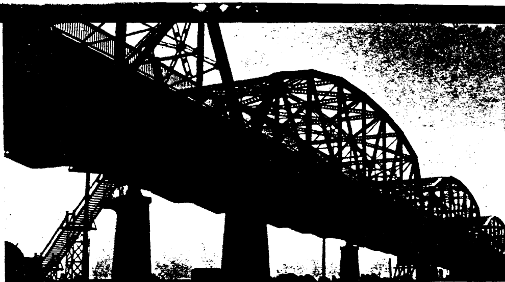
View of the Gibson R.R. Bridge showing some of its 3150 tons of structural steel. Corrosive industrial atmosphere pervades the area, severely testing the best of paint systems.
