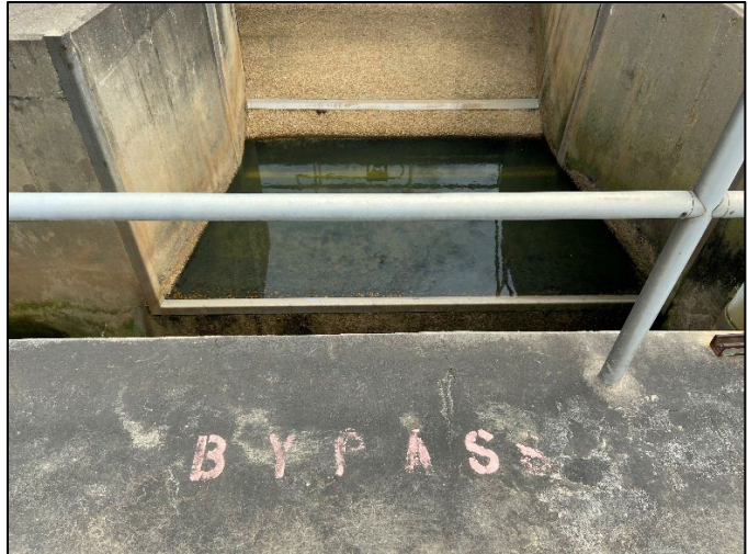
Photo 26: Bypass channel from storm cells.
