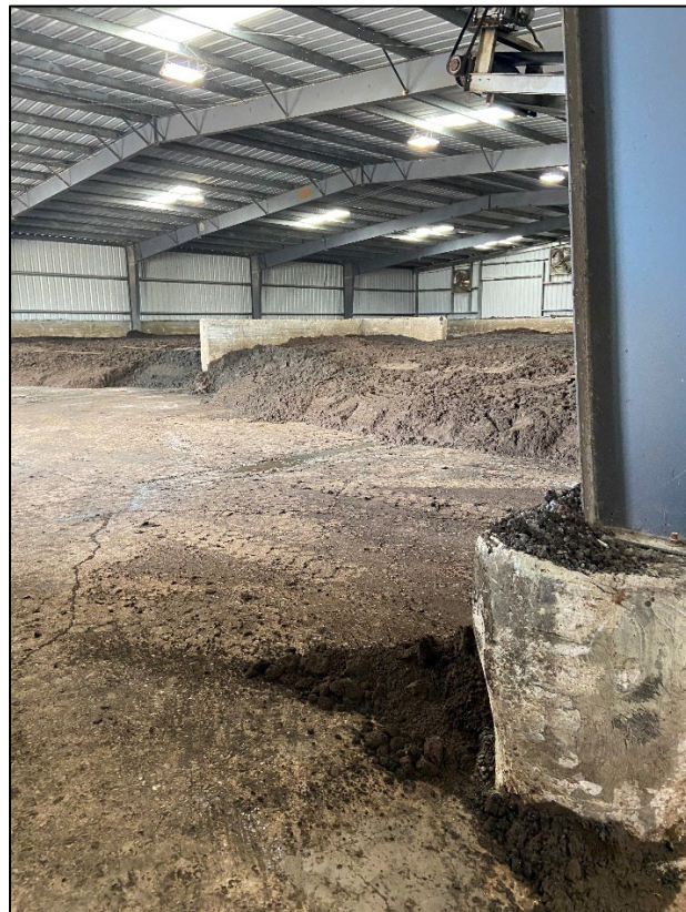
Photo 12: Sludge stockpile area.
