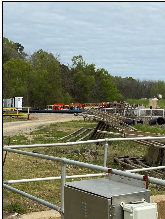
Photo 8: Rented bypass pumps (background).
