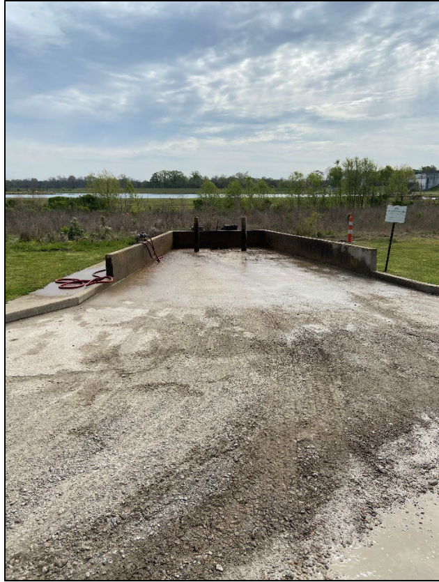
Photo 2: Septic hauler dumping station.
