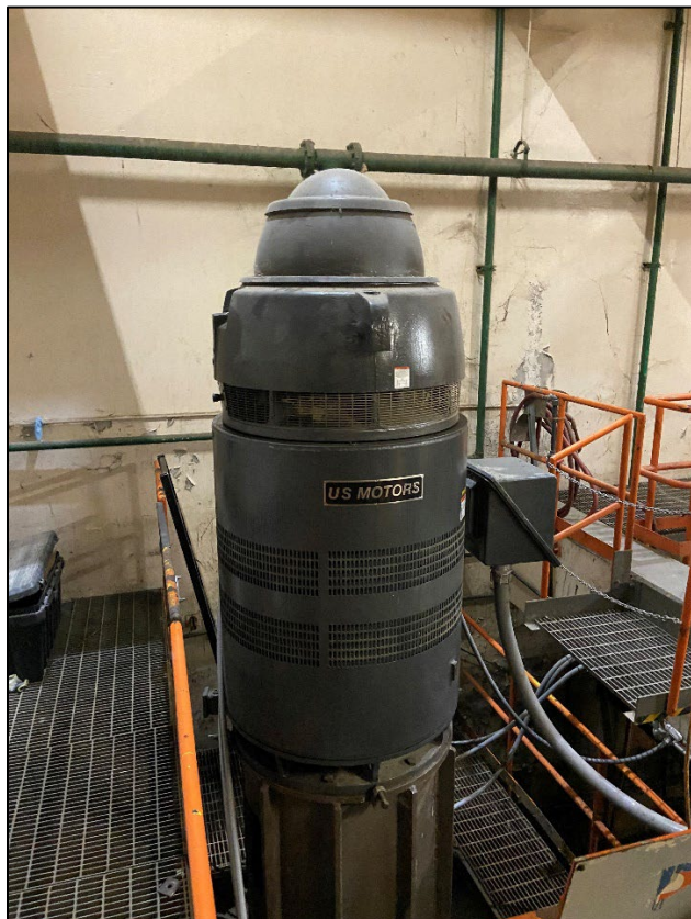
Photo 4: New motor on 45 MGD influent pump.
