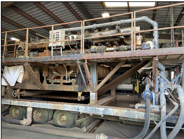
Photo 11: Sludge filter press.
