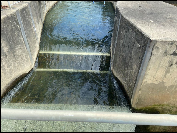
Photo 25: Effluent from mechanical plant.
