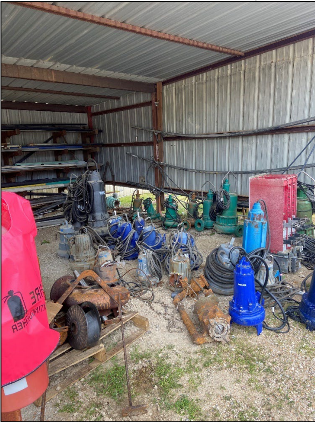
Photo 13: Replacement pump inventory.
