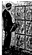
Cleaning Filter Elements with Portable Vacuum Cleaner
