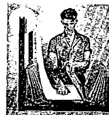
METHOD OF SERVICING Entire operation—unloading, refilling and replacing—consumes at most 3 minutes per unit. Useful life of filter medium varies from three to six months, depending on conditions
