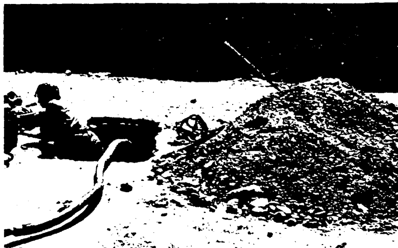
From the main, under the street, offset down two feet and into the basement, this lead service pipe is in one piece.
