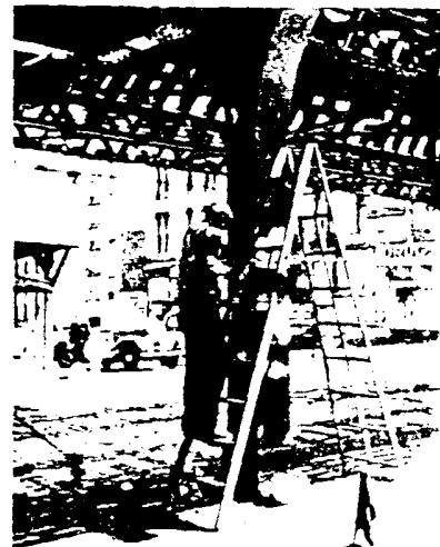
Painter at work applying red lead to a column of the 3rd Ave. El structure.
