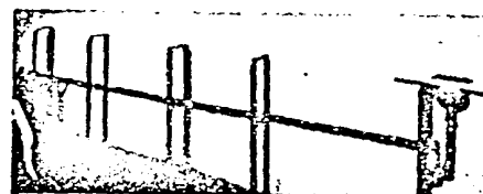
One of the many lead waste lines from the lead cup sinks in chemical laboratory tables installed in the new wing of the University of Arkansas Medical School.
