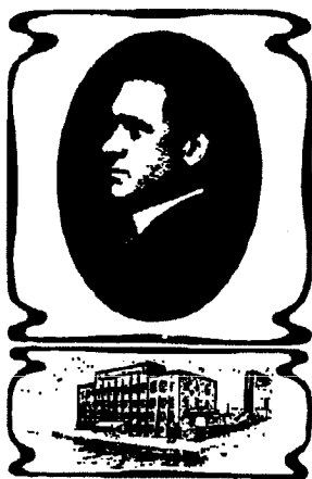
W. J. Lawson, Superintendent Newark Factory.
