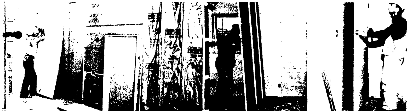
Face layer of Bestwall Gypsum Wallboard in Bestwall Hummer System A is applied with adhesive and nailed. First layer is only spot nailed.
