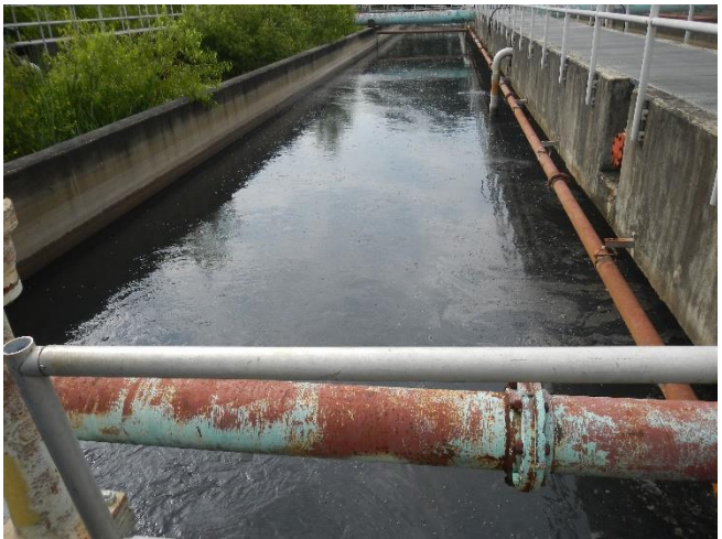
Photo 10: Digester Basin 8. Currently used for grit removal.
