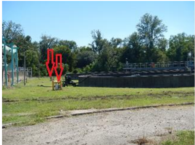
Photo 26: Ground water drawdown wells next to Clarifier Nos. 2 and 4. (red arrows)
