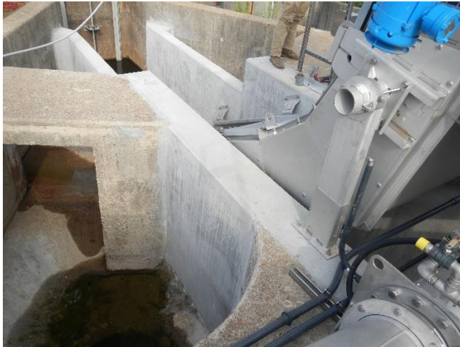
Photo 4: Bar screen and grit removal system under Construction.
