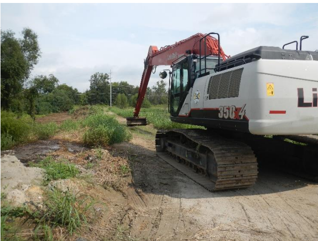
Photo 16: Sludge Lagoon 2 excavation work.
