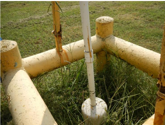
Photo 25: Piezometer located between Clarifier Nos. 3 and 4.
