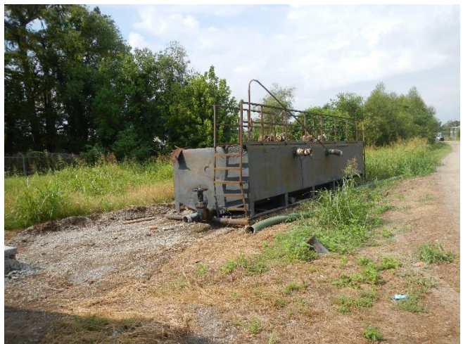
Photo 17: Tank outside sludge processing building planned for sludge processing.
