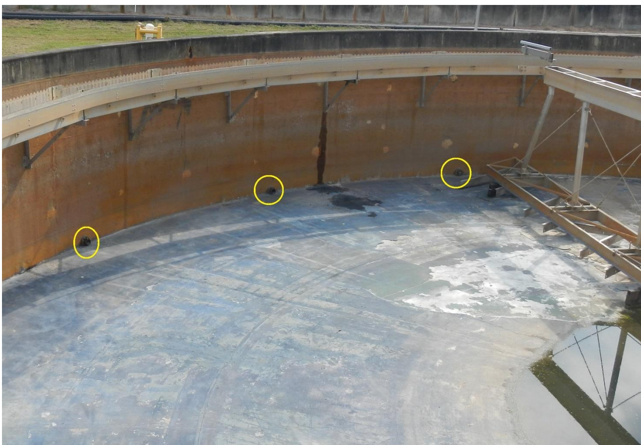
Photo 29: Clarifier GW relief valves (yellow circles).
