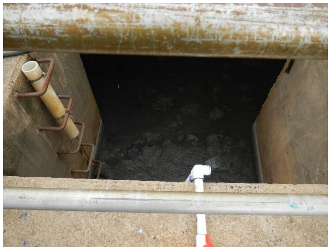
Photo 21: Effluent well.
