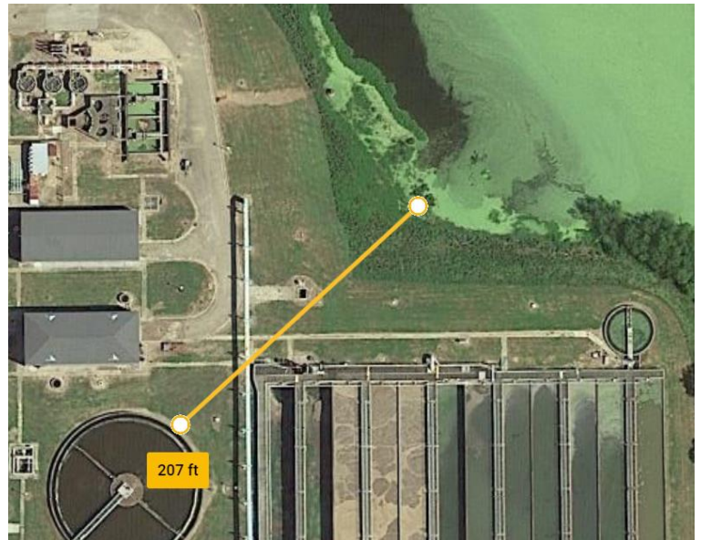
Photo 24: Google Earth screenshot of slough, clarifiers and Aerator/Digester Basins.
