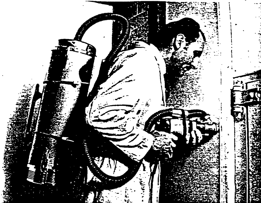
44 Portable suction equipment for use when drilling asbestos insulation board. Photo: Owen Lawrence, London.
