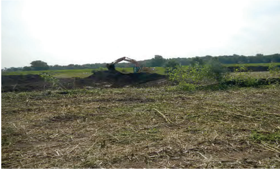
Photo 1. Construction of the north Basin
