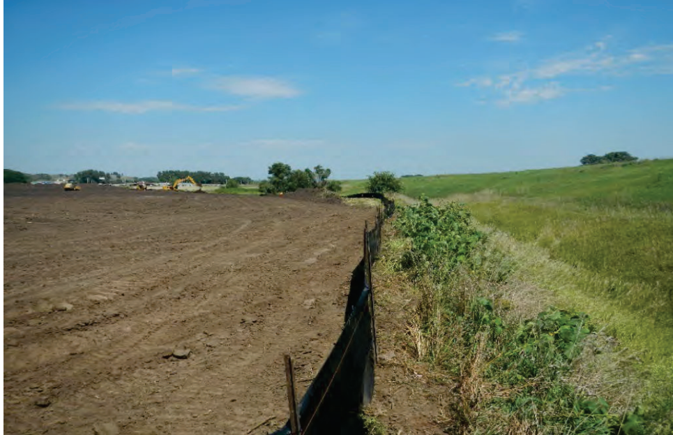
Photo 4, Contractor installing the silt fence along the east perimeter
