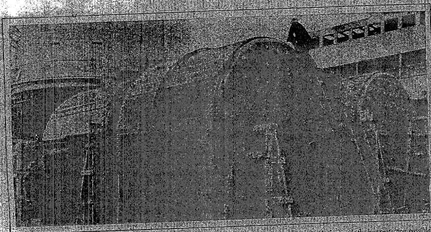
Metal of boilers needs the best protection possible for the boiler plate, after painting, is covered with asbestos and is made suitable for inspection, preventing the boiler from rusting and cracking.
